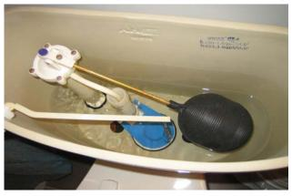
First shut off the water valve underneath the toilet by turning all the way to the right. Then flush the toilet - to keep the top tank empty. To remove the flapper valve, pull the rubber hinges away and then up from the central cylinder. Afterwards you will need to pull the rubber string through the plastic that connects to the flush handle (see the chain in the above picture). This will release the flapper valve completely.
