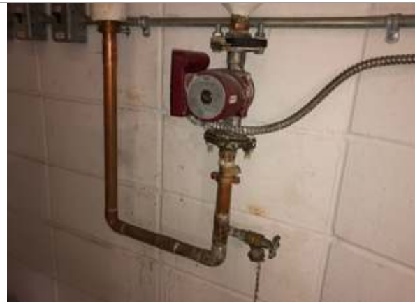
Photograph 100 Recirculating pump
