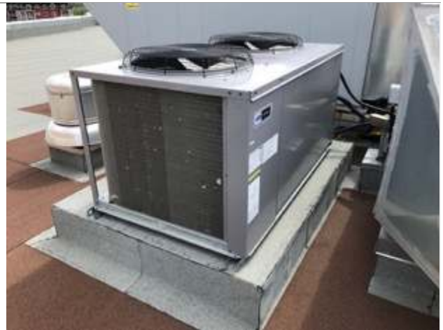
Photograph 117 Condensing unit
