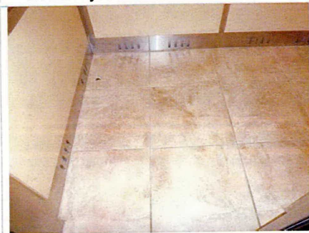
Elevator cab interior
