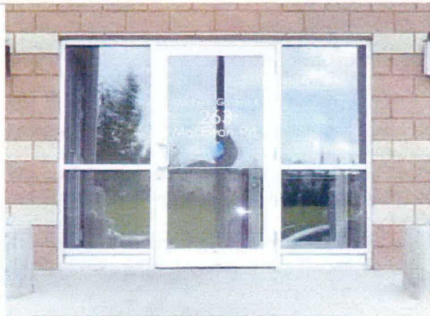
Front entrance door
