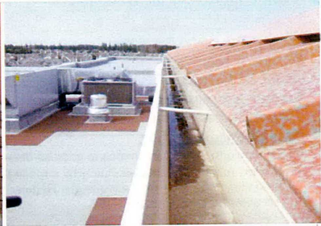
Eavestrough clear of debris
