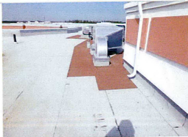
Downspout draining onto SBS membrane roofing
