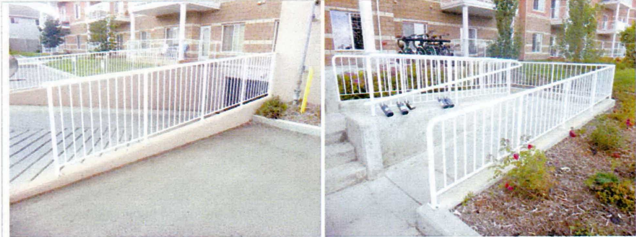
Metal railings installed on retaining walls
