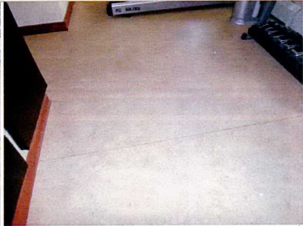
Linoleum installed in fitness room
