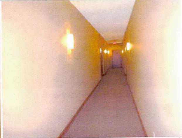
Smooth paint finish on walls
