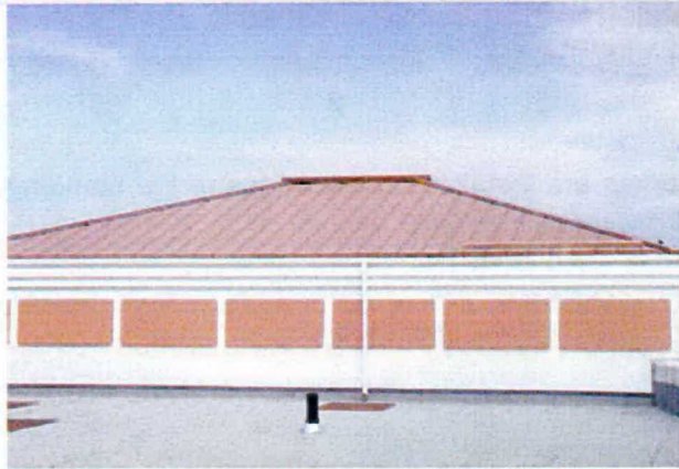
Overview of standing seam metal roof
