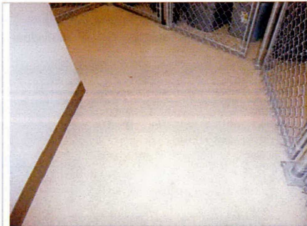
Vinyl tiles in storage room
