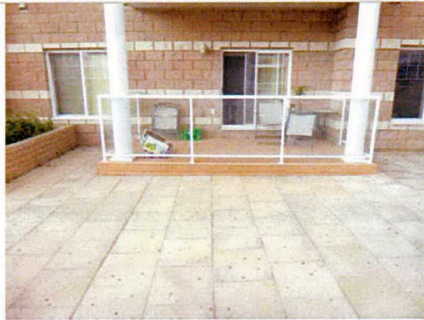
Composite wood deck with glass railings
