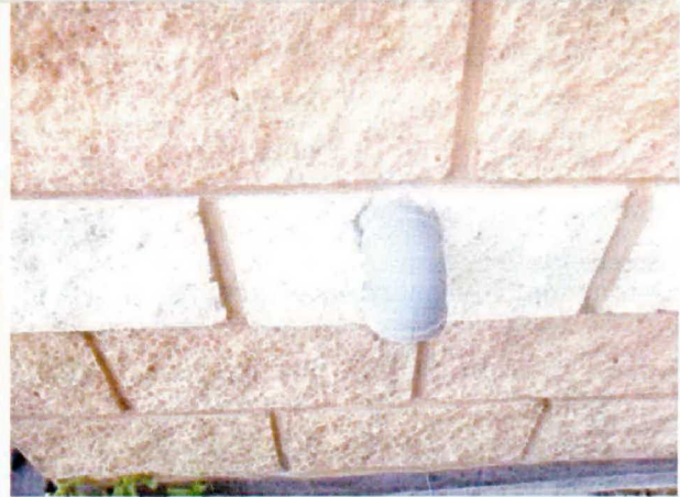
Sealant around wall penetration
