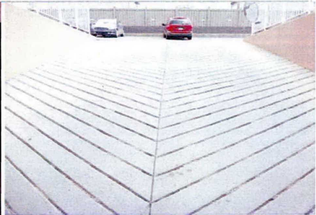
Poured concrete ramp
