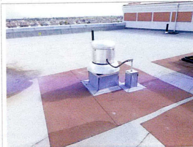
Protective layer of membrane on traffic areas
