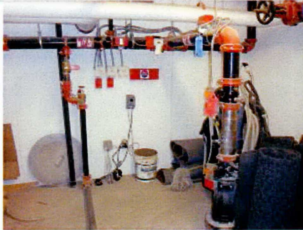
Main sprinkler connection
