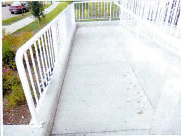
Concrete ramp adjacent to steps
