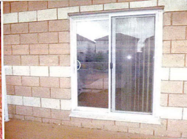
Exterior of horizontal slider patio door
