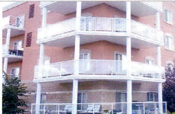
Glass railings, metal fascia and column cladding
