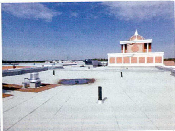
SBS roof and copper shingled architectural feature
