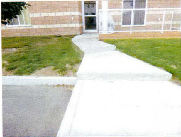
Concrete walkway leading to stairwell exit
