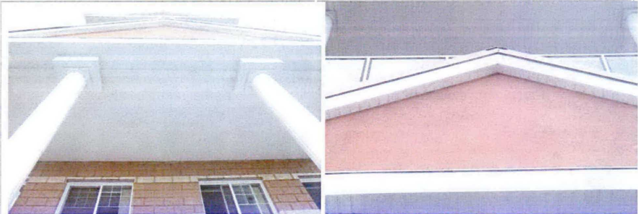
Soffit on underside of canopy
