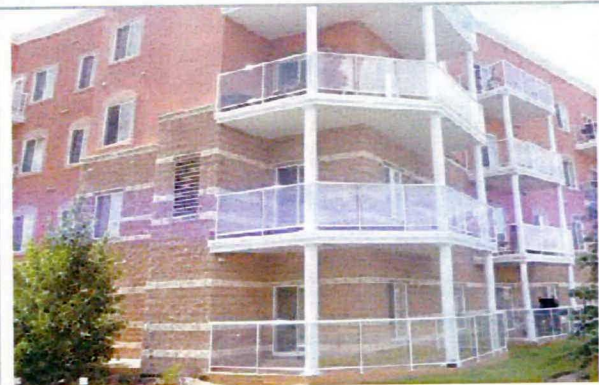
Architectural block veneer
