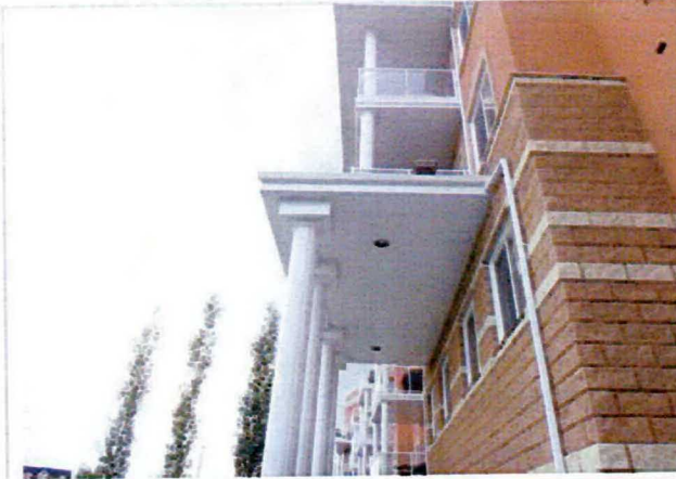
Eavestrough on edge of canopy roof
