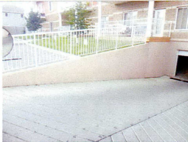
Concrete retaining wall at parkade ramp
