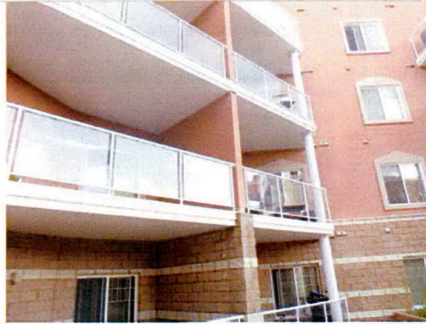
Stucco clad privacy walls
