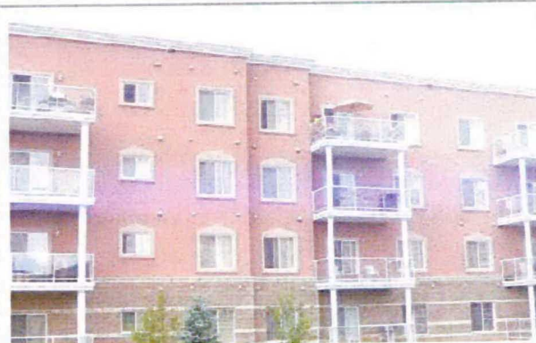
Stucco with EIFS trim around windows and decorative cornice
