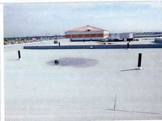
Overview of SBS roof area
