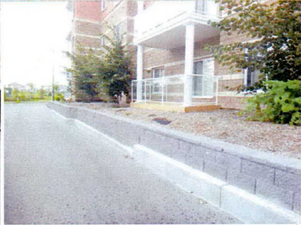
Allan block retaining wall
