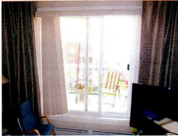
Interior of horizontal slider patio door
