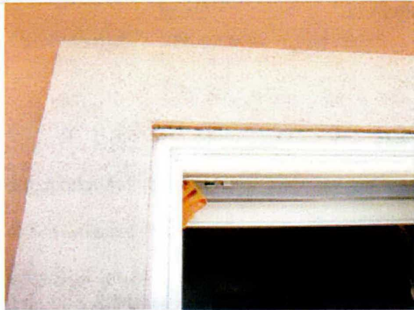
Sealant around window
