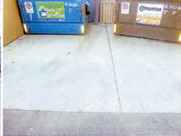
Poured concrete pad
