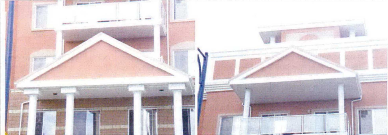
Prefinished metal fascia installed on the edge of canopy roofs
