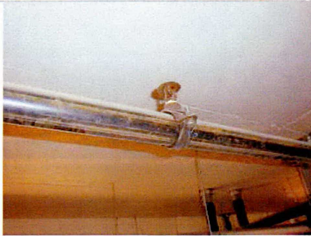
Main sprinkler connection
