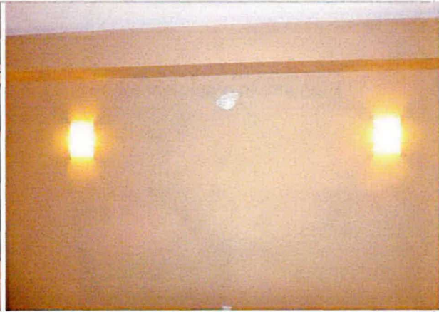
Wall and emergency lighting
